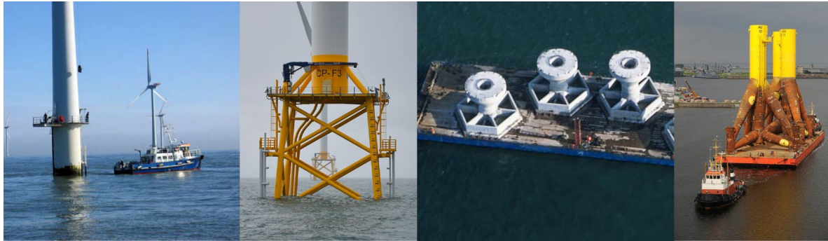
FIG. 1. (Color online) Different foundation types. From the left, Monopile (Horns Reef 1), Jacket (Thornton Bank), concrete (Nysted), and tripod (Alpha Ventus) are shown.
